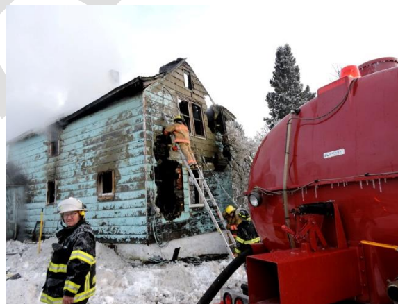
Fire fighters searching the interior of Fulton structure for hotspots following fire (Source: Graham Jaehnig, Daily Mining Gazette)
