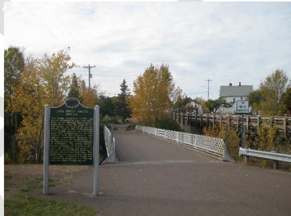
Eagle River Bridge (Source: Richie Diesterheft )
