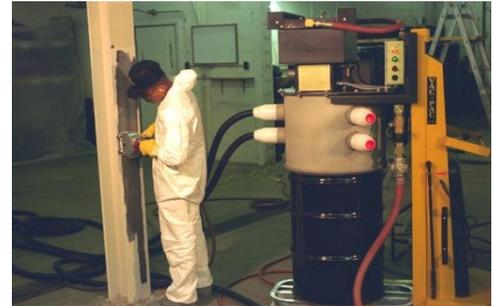
*Worker is using the roto-peen (scabblor) attachment; VAC-PAC collection system shown with 55 gal drum.*
